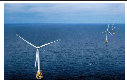
Offshore Wind Turbine
