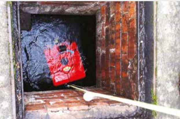
▲ The ROV deployed via the access hatch
