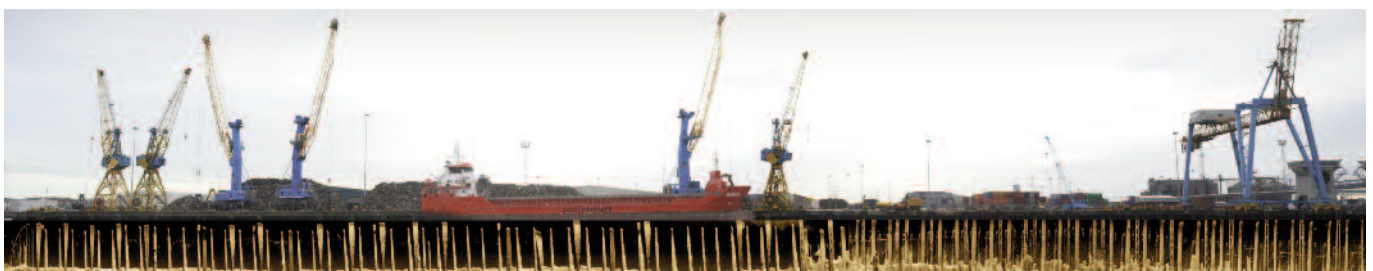
Image showing Newcastle docks, visible targets from the StarFish 990F data includes the dock struts and supports.
