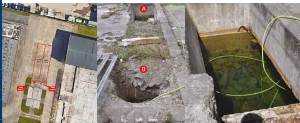
Images courtesy of CDMS Sub Surface Engineering
